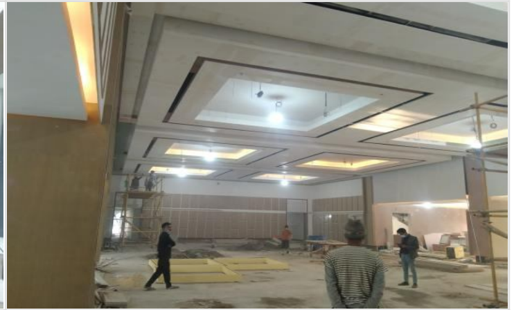
Interior work on 31-01-22
