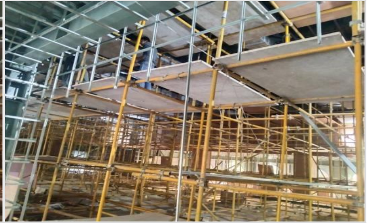
Interior ceiling on 05-01-22
