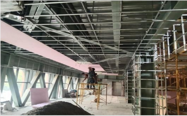
First floor ceiling work on 05-01-22
