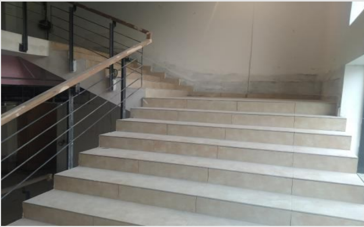
Tiles work on 31-01-22
